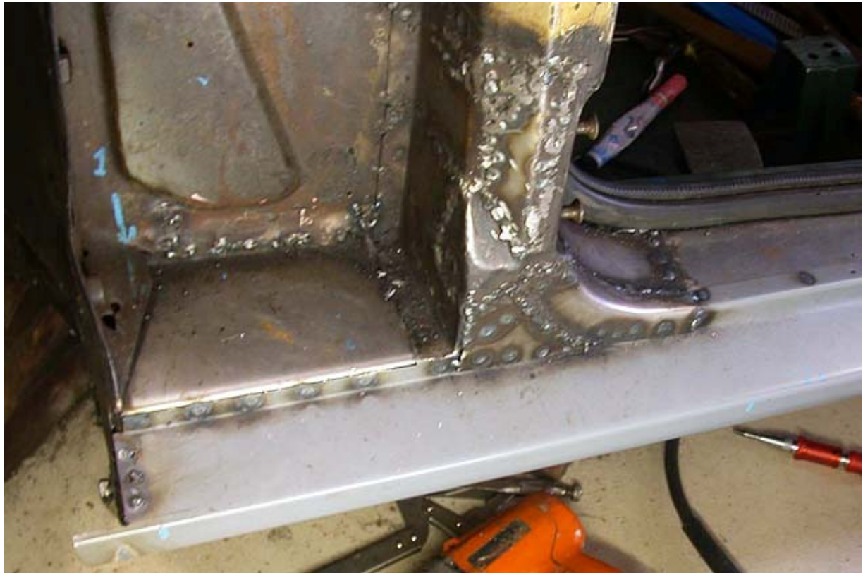
Figure 8 Finalising the A pillar fabrication
