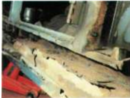
General view of rust in offside side-beam.
